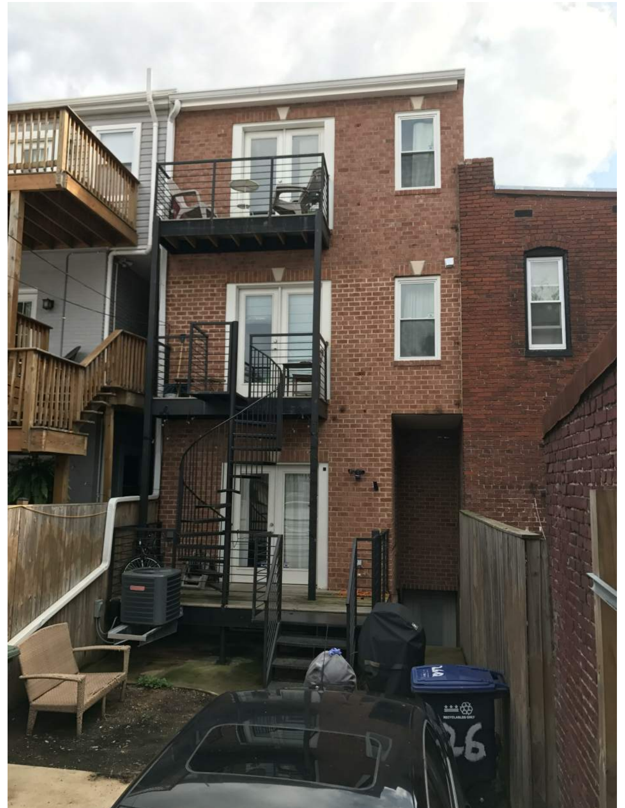
② EXISTING CONDITIONS PHOTOGRAPH - NORTH ELEVATION 12" = 1'-0"
