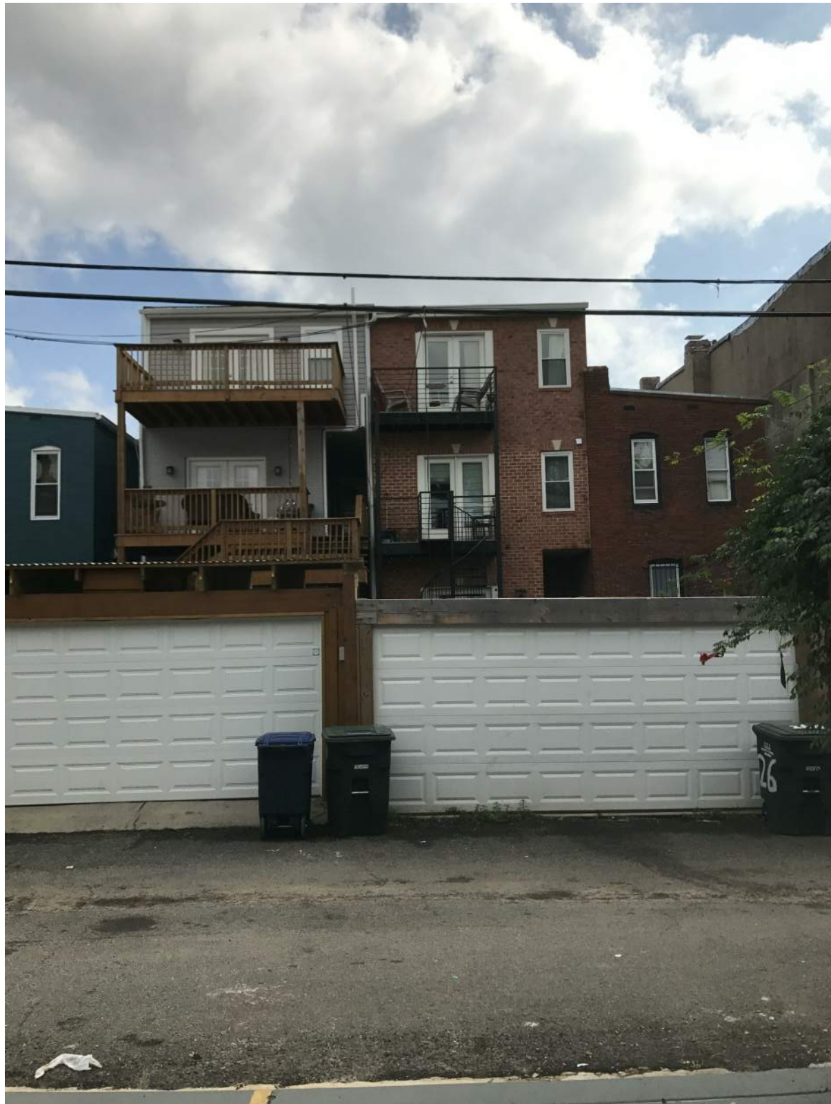
① EXISTING CONDITIONS PHOTOGRAPH - ALLEY ELEVATION 12" = 1'-0"
